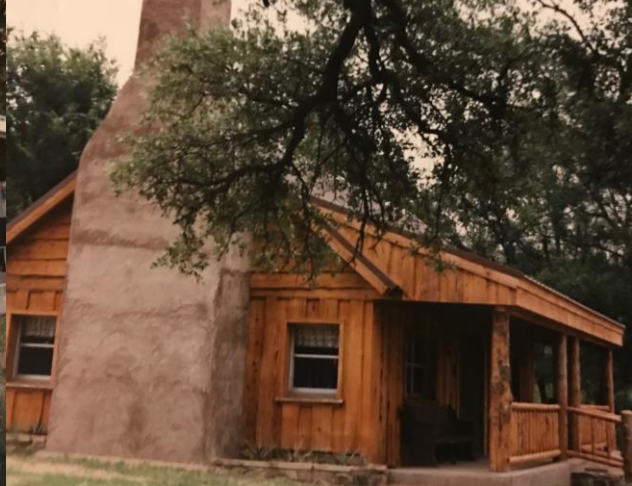
Bunk House after Improvements
