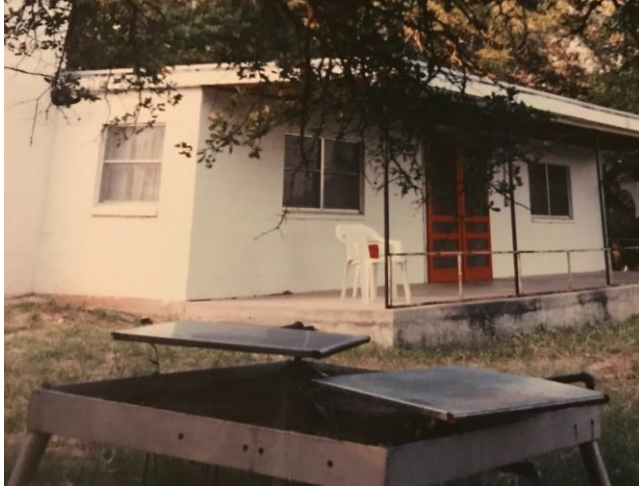
Bunk House before Improvements
